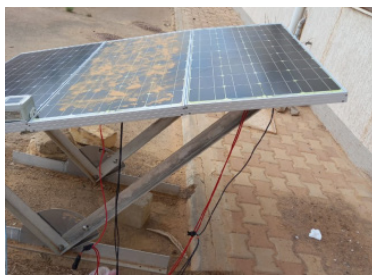
Figure 3. Installing the solar panels
